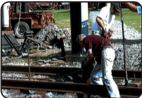
Dave helping lay tracks at the yard.
